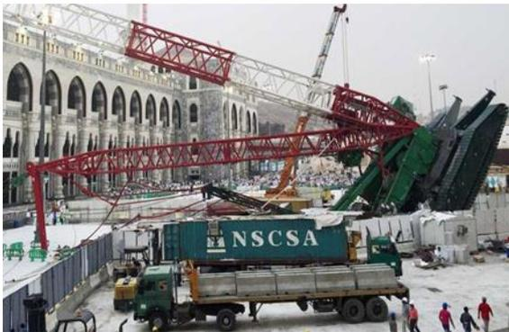
Gambar 57. *Crawler crane* Roboh
